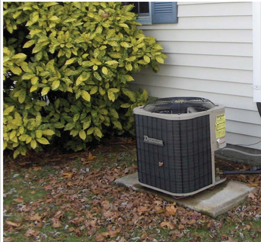
Heat pumps use electricity to extract heat from the ground or air and use it to heat or cool buildings. Using one unit of electricity moves about three units of heat.
