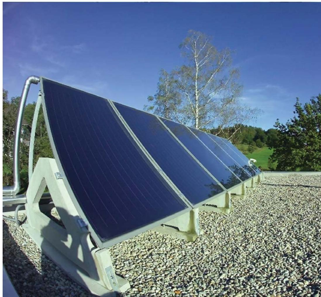
Energy from sunlight can to some extent replace fuels to heat water and buildings if solar collectors are used.
