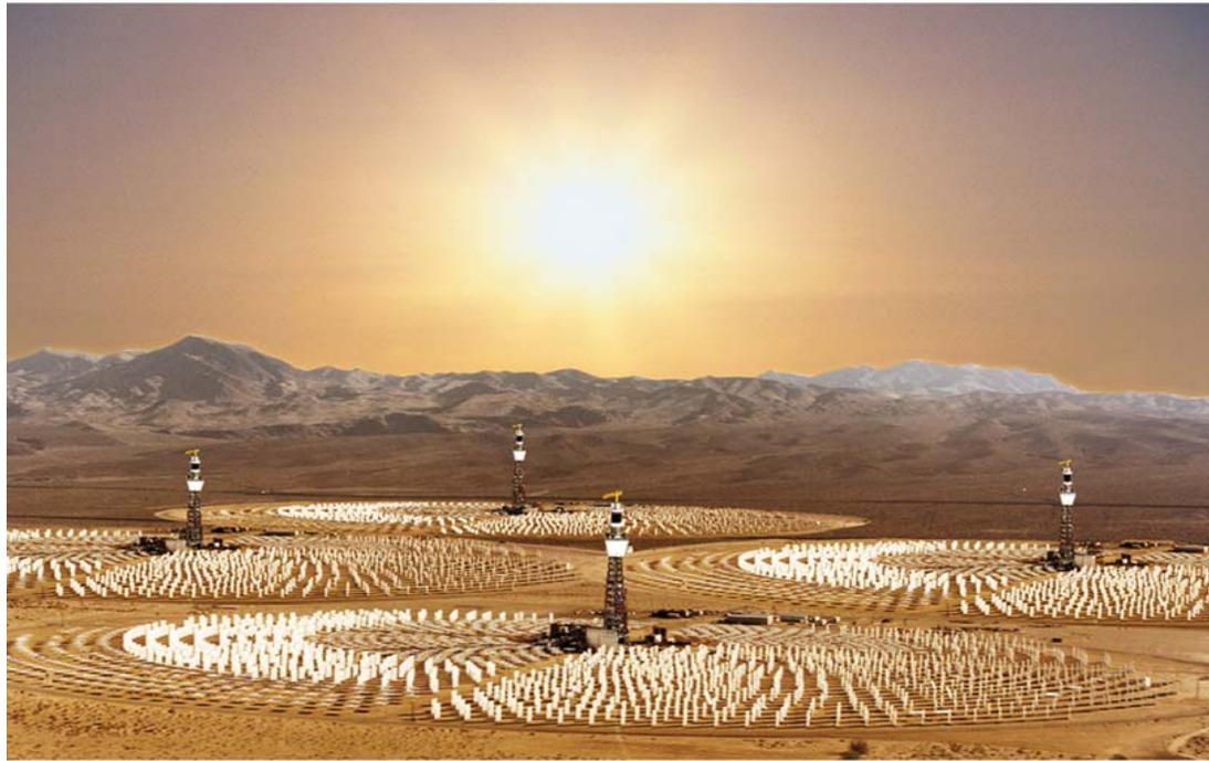
Concentrating sunlight with mirrors produces heat similar to burning fuel. High levels of radiance are needed to run the generate electricity sufficiently.
