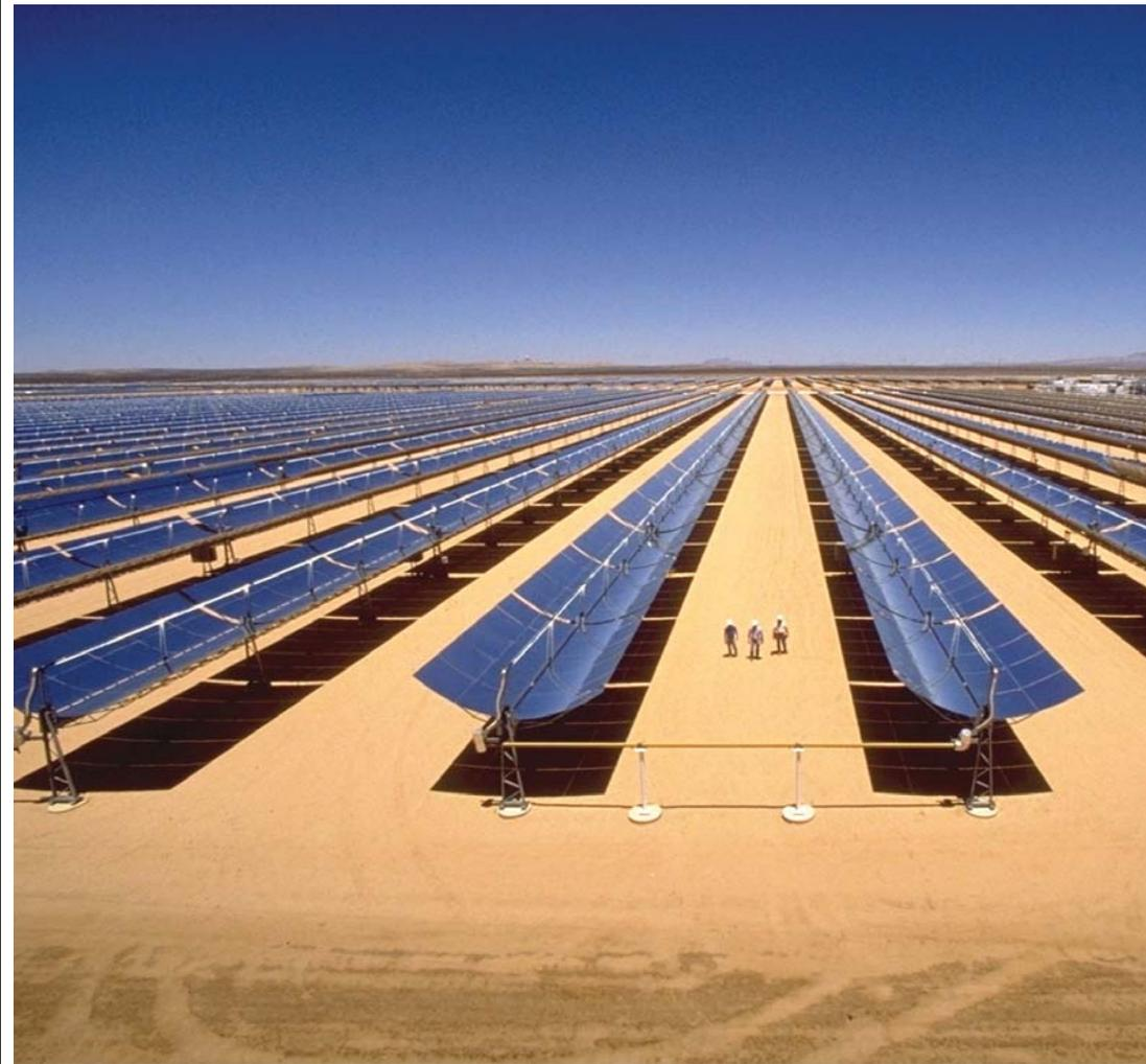
Heat and steam generation for processes in e.g. chemical industry could be done using concentrated solar power instead of burning fuels.
